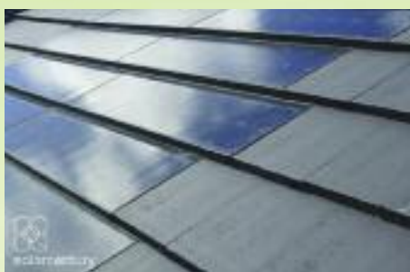
Close-up of integrated roof-top solar panels.
